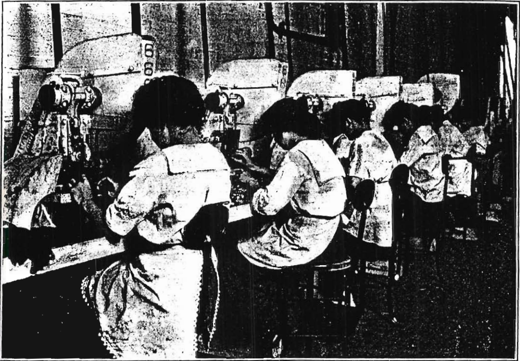
WOMEN OPERATING PUNCH PRESSES IN WAGNER FACTORY Note the white finish on the machines and the stools with back rests
